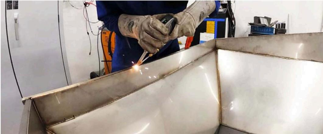
Figure 8. Handheld laser beam welding on the funnel
